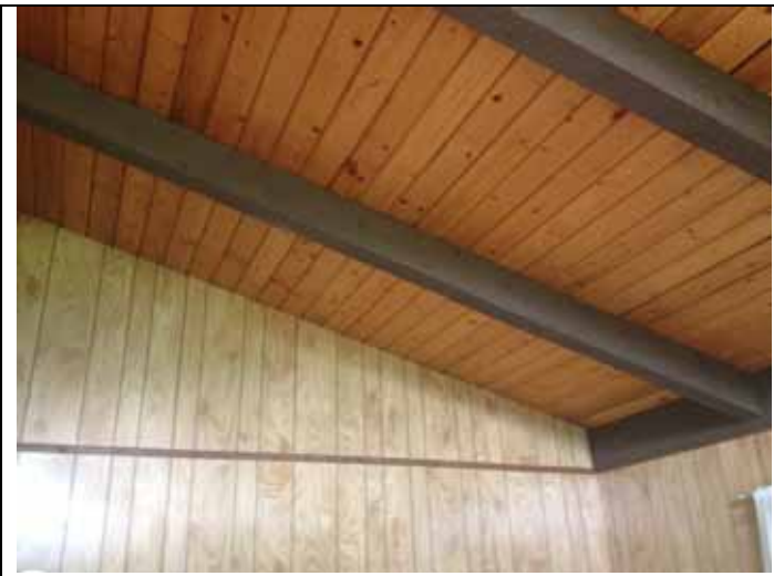
17. View of the ceiling and walls.
