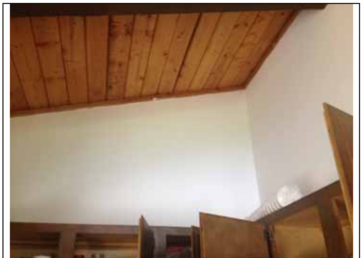
22. View of the kitchen ceiling and walls.
