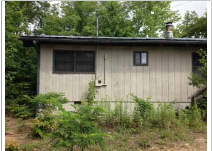
14. View of the south side of the home.
