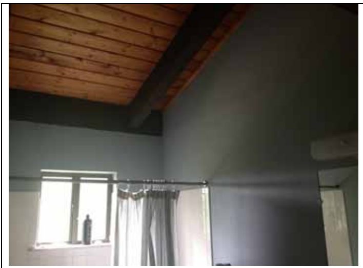
21. View of the walls in the bathroom.
