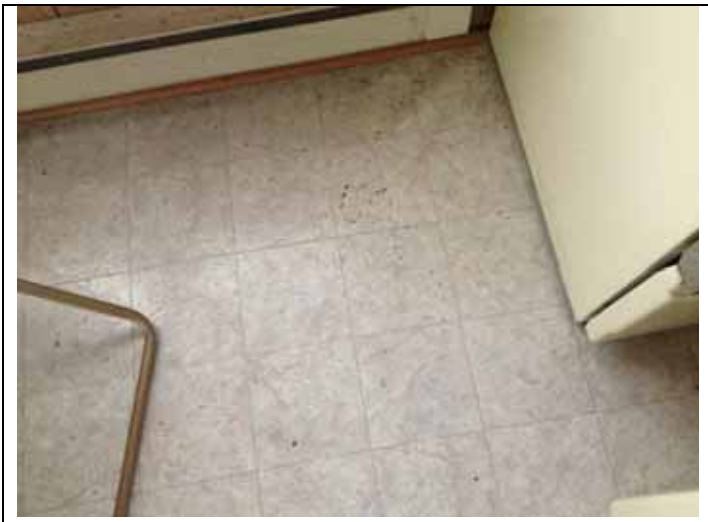
23. View of the floor in the kitchen.
