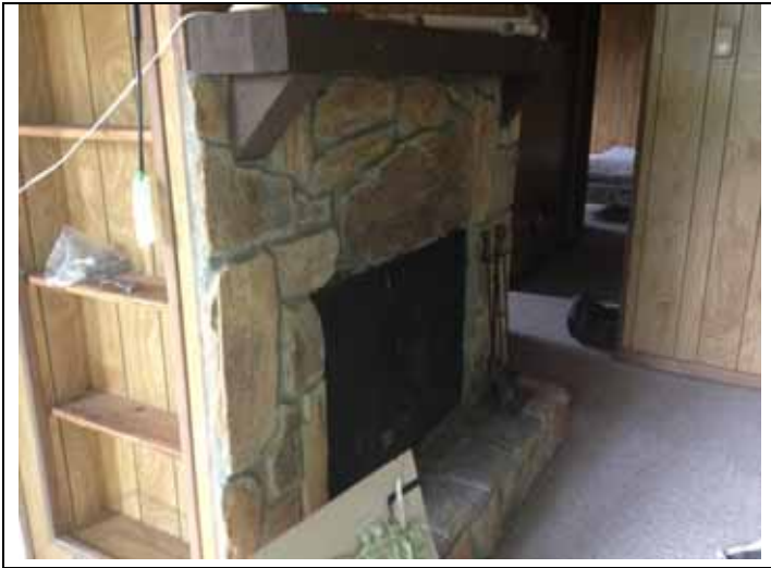
19. View of the fireplace.
