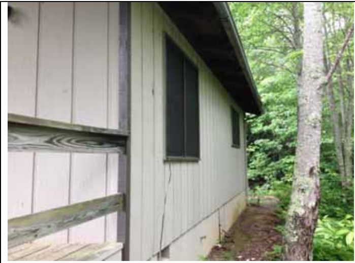
13. View of the north side of the home.
